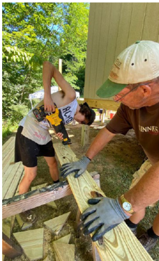
Luke Jordan (left) uses a sawzall.
