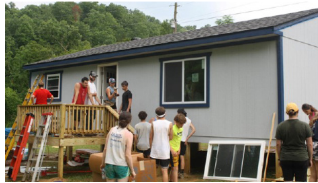
Home builders in progress.
